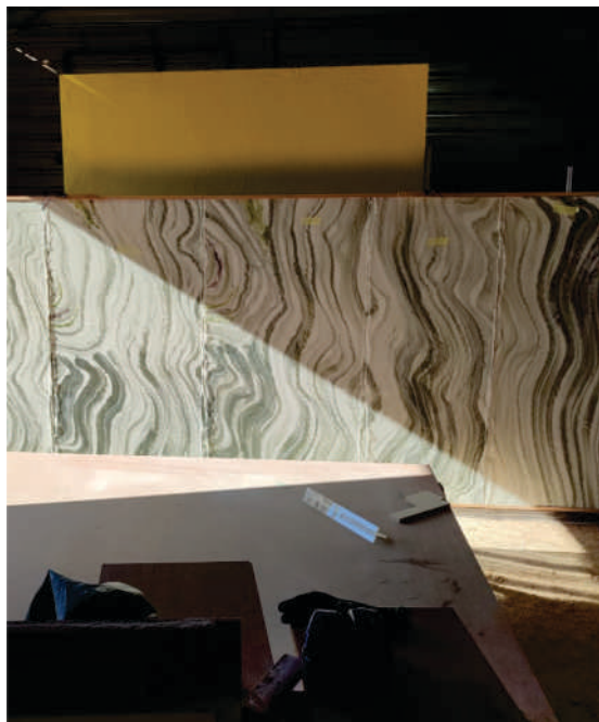
ALIGNING PATTERNS BETWEEN PANELS
