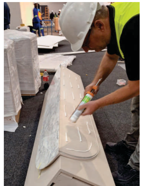
EVENLY-APPLIED EPOXY USED TO FIX PANELS DIRECT TO SURFACES
