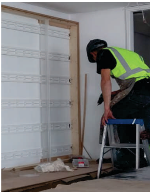
EXAMPLE OF PERSPEX COLUMN PROVIDING SUPPORT BEHIND JOIN LINES
