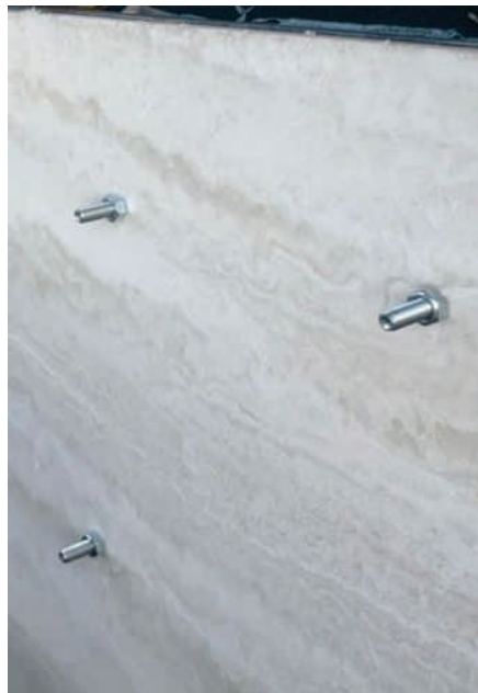
LIGHTWEIGHT LOADS CAN BE FIXED DIRECTLY INTO LUMOSTONE PANELS
